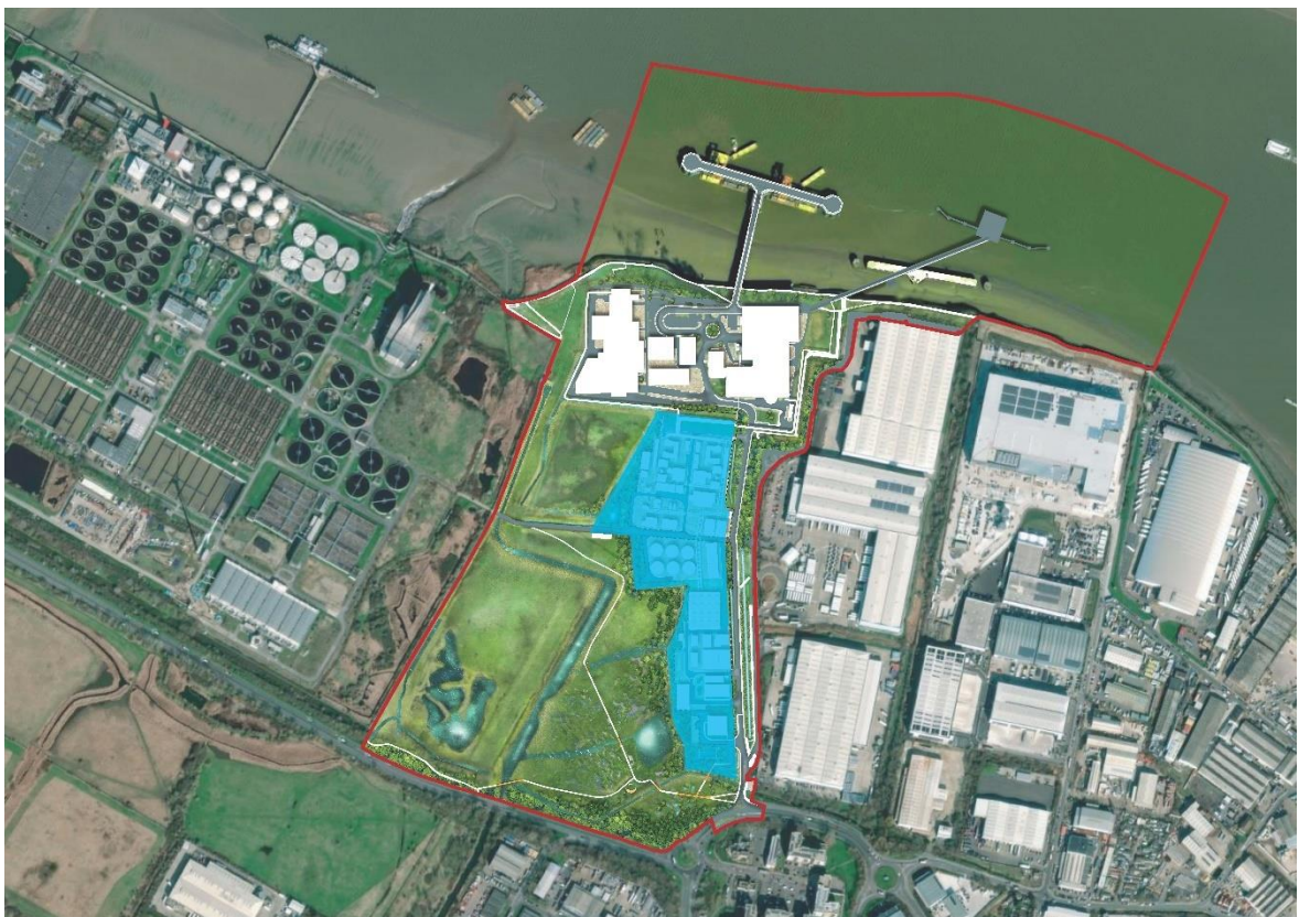
Figure 6 Carbon Capture Facility (CCF) Area
